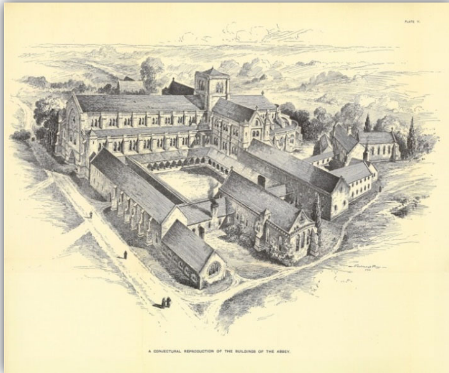
Figure 37: 'A Conjectural reproduction of the buildings of [Beaulieu] Abbey' illustration (Brakspear, in Fowler, 1911)
